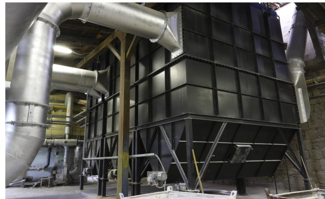
Dust collector IKV 3,4-200-278-PT Capacity 18.000 m 3 /h (250 °C)
