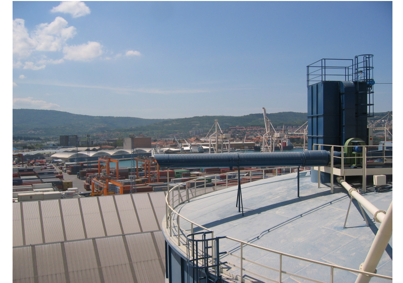
Dust collector FVS 3,0-144-176 Capacity 15.000 m 3 /h
