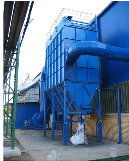
Dust collector IKV 4,0-240-387 Capacity 35.000 m 3 /h
