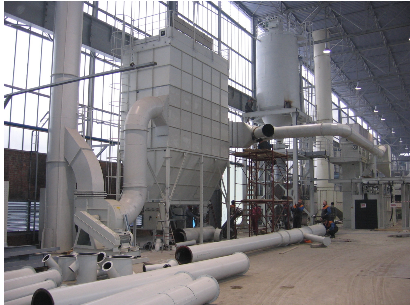
Dust collector IKV 4,0-240-387 Capacity 35.000 m 3 /h
